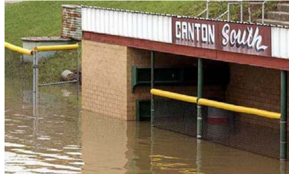
Canton South High School baseball dugout, Nimishillen Creek overflowed its banks
