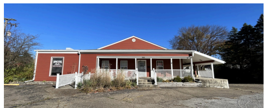
Vacant Building on Lincoln Way
