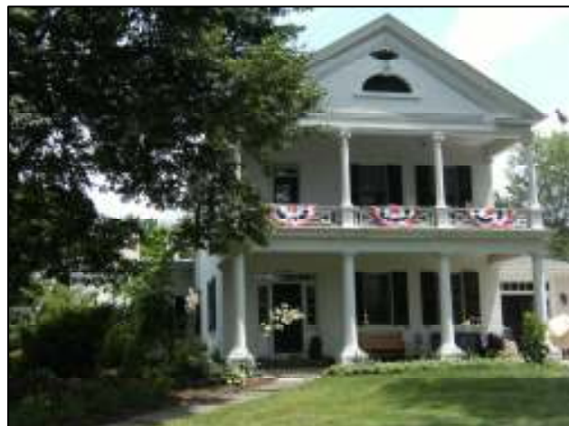
Historic Housing Stock/Adaptive Reuse Example Source: Fulton House on Pleasant Hill website
