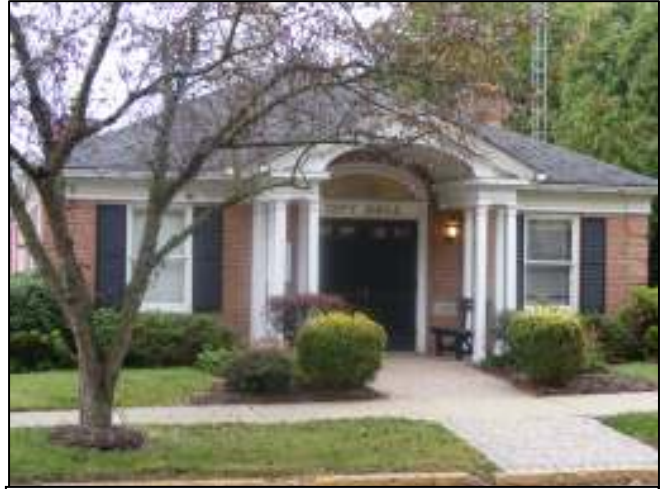
Canal Fulton City Hall Source: SCRPC
