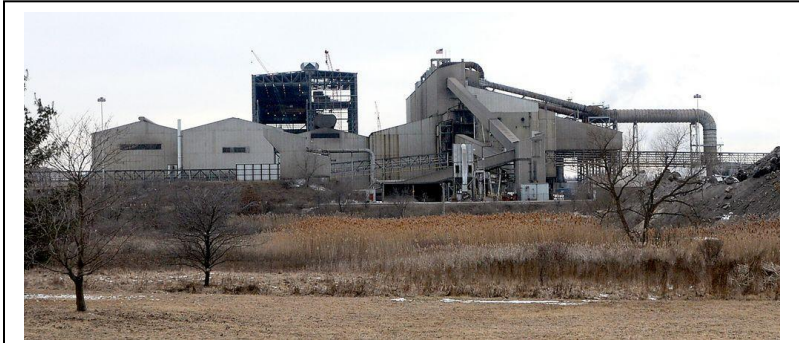
The Timken Company's Faircrest Plant located in Perry Township Source: Canton Repository
