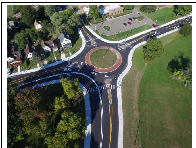
12 th Street Roundabout Source: SCATS
