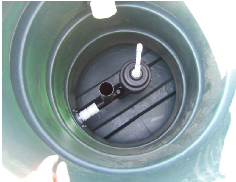
Figure 6. Dosing siphon - internal view
