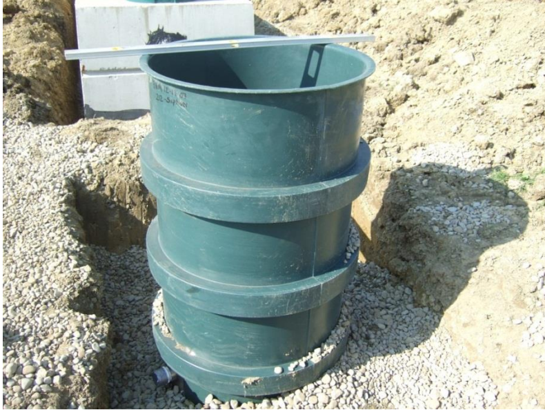
Figure 5. Dosing siphon - external view
