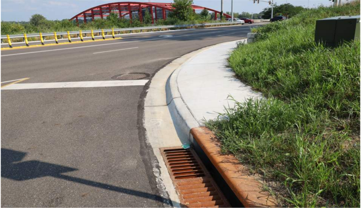
Location: Strip Ave at southern Walmart Driveway looking south Observation: The sidewalk ends at a location without a curb ramp and crosswalk.
